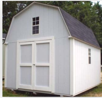
Gambrel Style Roof- Lots of Overhead Storage
